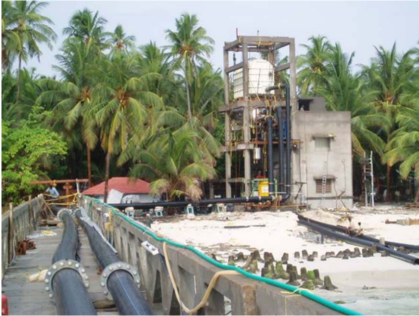
Fig. 9.5. A picture of the 100,000 l/day capacity LTTD plant in operation at Kavaratti (Kathirolu et al., 2006).
