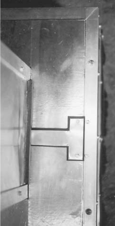
FIGURE 6-25. T-shaped gap cover for lower access panels.
