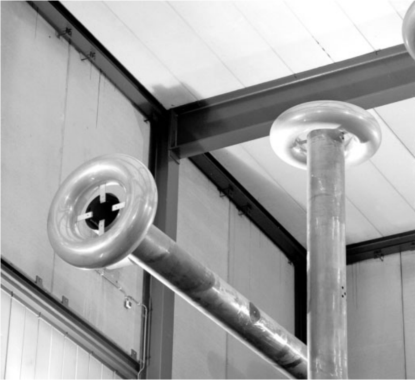
Figure 10.18 The spark gap of KEMA's synthetic test facility can be triggered with an accuracy of microseconds (courtesy of KEMA)
