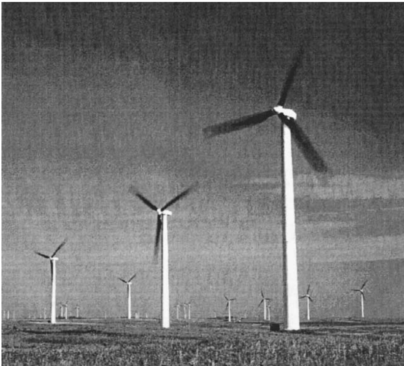
Figure 9.6 Wind farm in the midwestern United States. (Courtesy of Enron Corp.)
